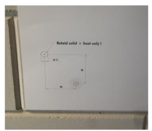
2. On the left bottom-side of the back plate you will find an eye. Use an awl or screwdriver to puncture the sealing plug. Run the whole cable of the heating element through the hole.
